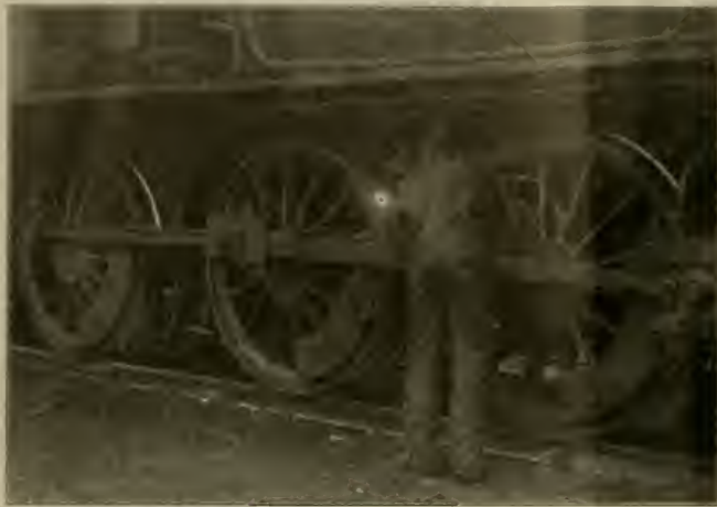
BUILDING UP FLAT SPOTS ON LOCOMOTIVE DRIVERS.
